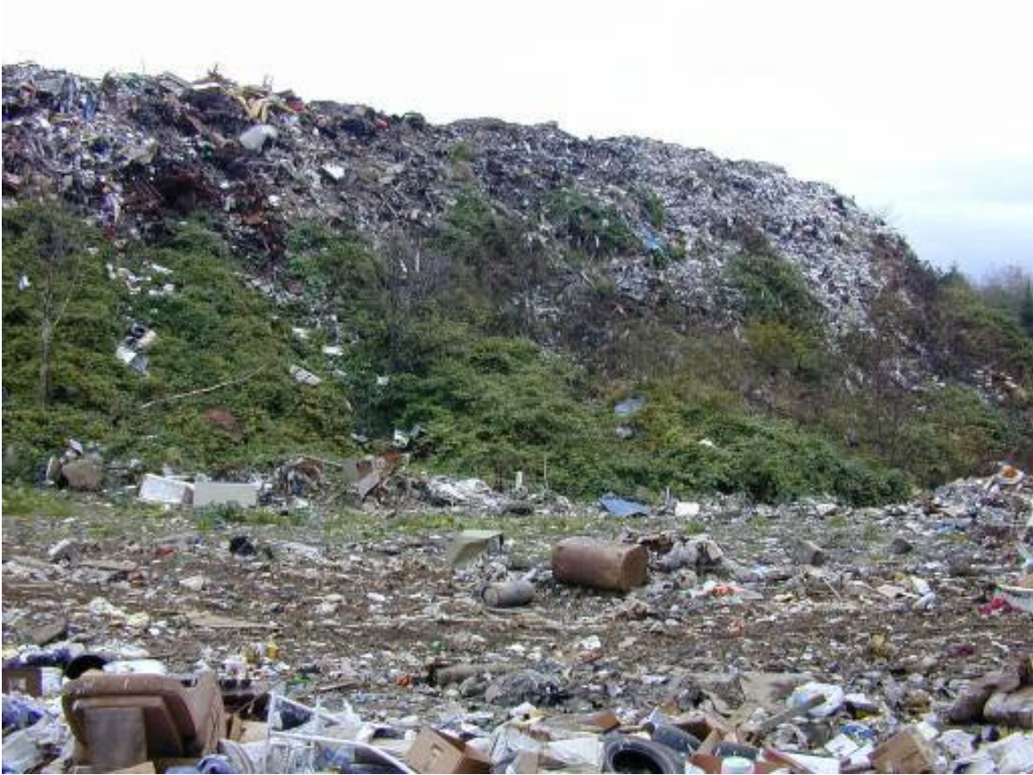
Figure 3. Photo showing a general view of the Warmhouse Beach Open Dump.
