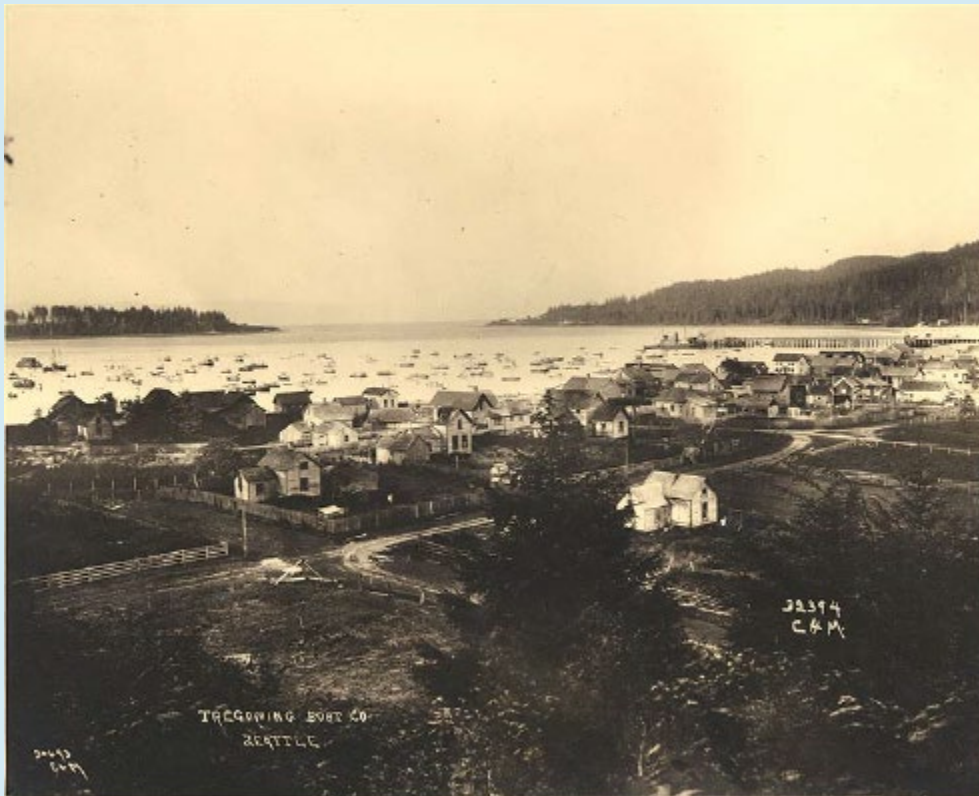
Figure 4: Photo of Neah Bay looking northeast towards Wa'adah Island and Agency Creek. Photo taken in 1915 by Asahel Curtis (Fitzpatrick 2006).
